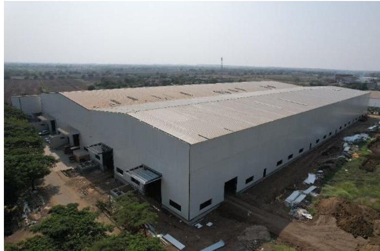
New Assembly Lines
