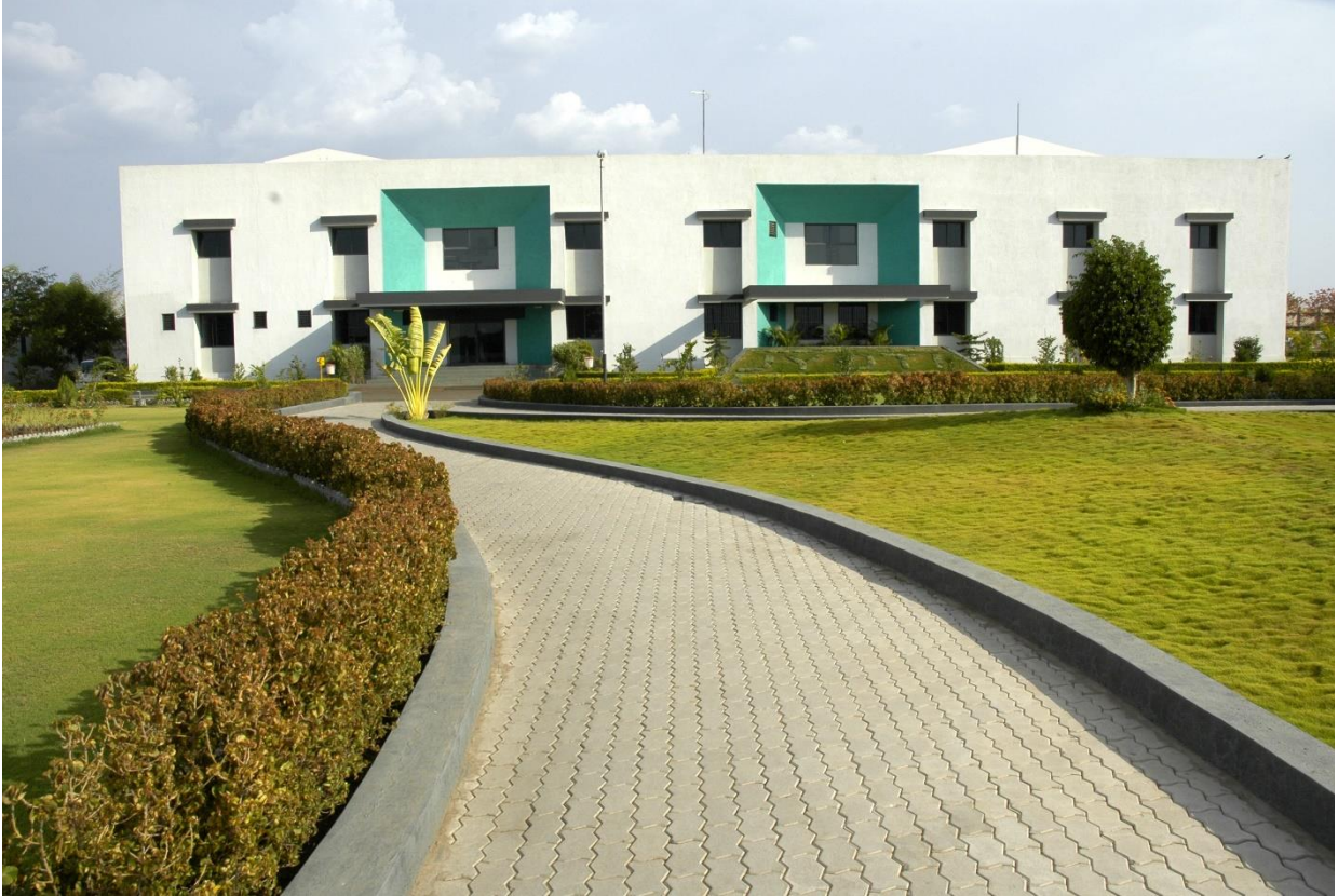
Machine Shop Building
